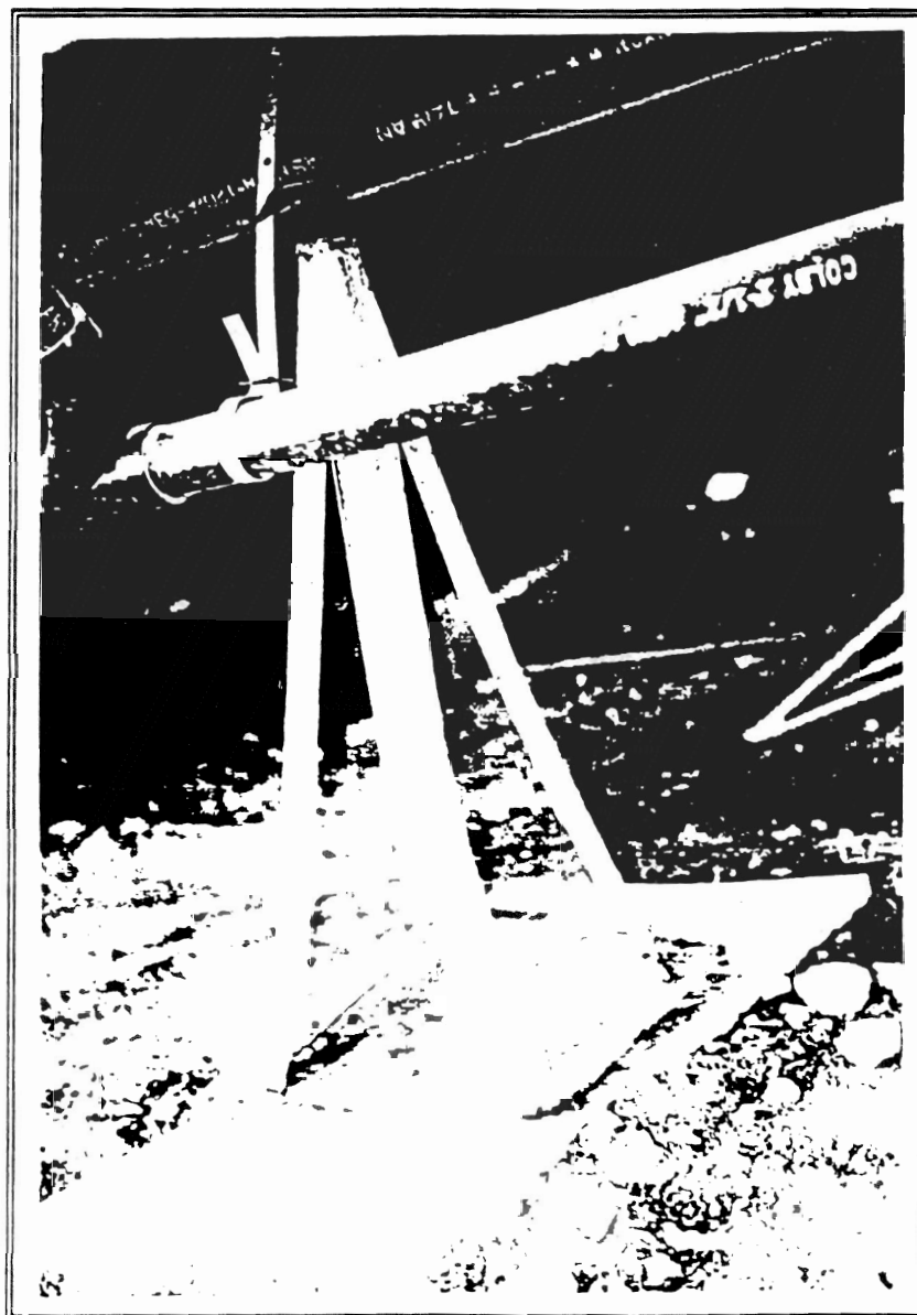
ILLUSTRATION 1 Chassis beam shifted off steel pier
